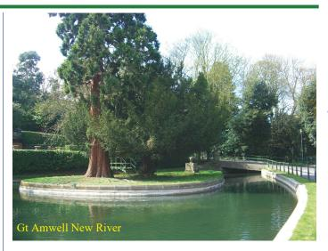
The New River was opened in 1613, following the land contours so that gravity carried the water all the way to the Clerkenwell area of London. In 1620 a half mile extension was dug to supplement the supply by taking water from the nearby River Lea. After 400 years, the man-made New River still takes fresh water to the citizens of London; it is now operated by Thames Water.
